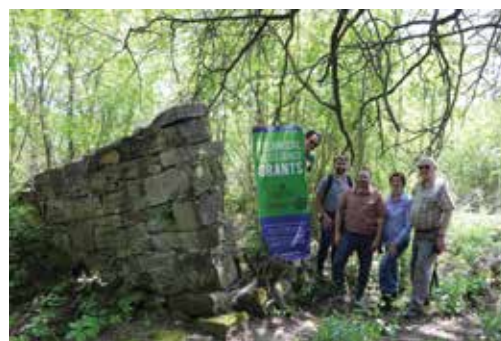
◀ Team members from John G. Waite Associates, Architects, visit the remaining wall of the Smith's Forge in the Lower Town.
